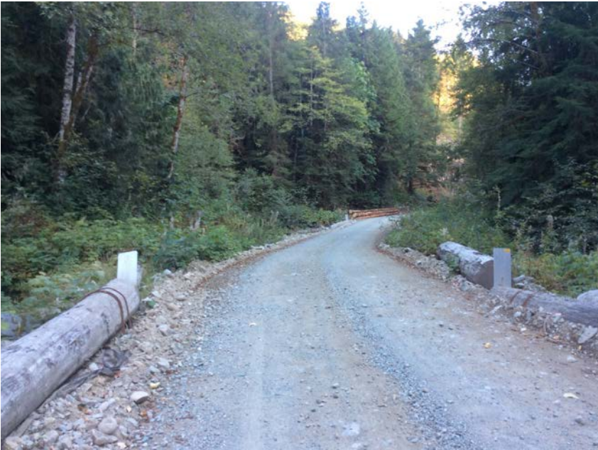
Left approach viewed from bridge
