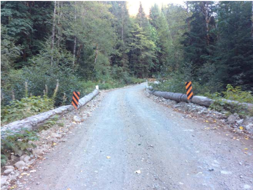
Approach from Right Bank when facing downstream
