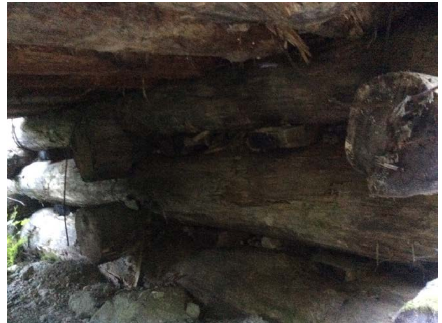
Right Bank Abutment when facing downstream
