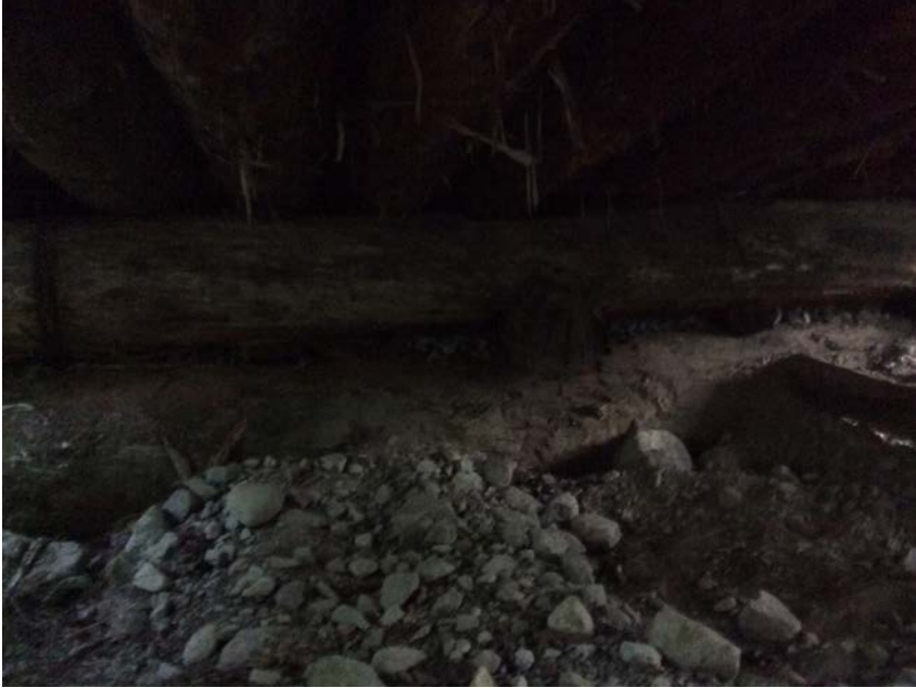
Left Bank Abutment when facing downstream
