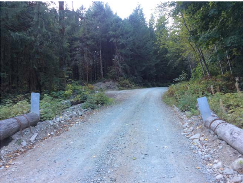
Right approach viewed from bridge
